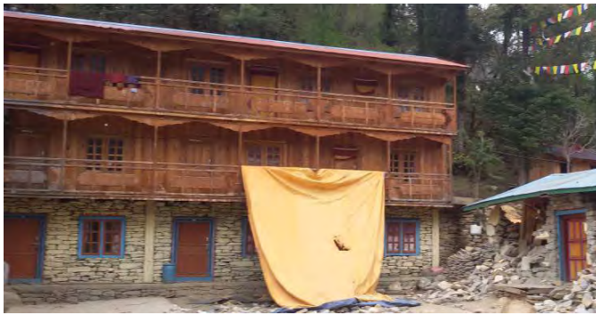
a) Mixed material and structural systems (RC frame, timber and stone in bottom storey and timber in upper storey (source: Subash)
