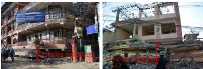
Photo 2: Soft story failure (lost their lower 2 and 4 stories) of buildings in Gongabu
