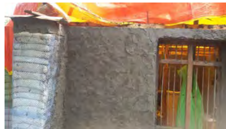
Figure 20: Plastic mesh and cement plaster (Good Earth Nepal, 2015)
