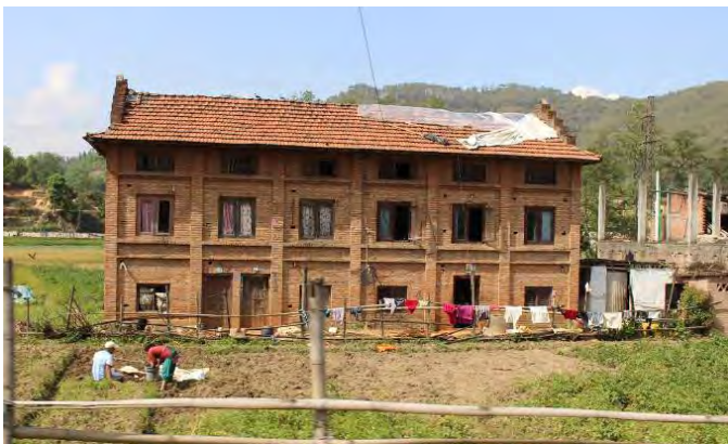
a) A brick in mud mortar with timber floor and timber roof structure, Kathmandu valley
