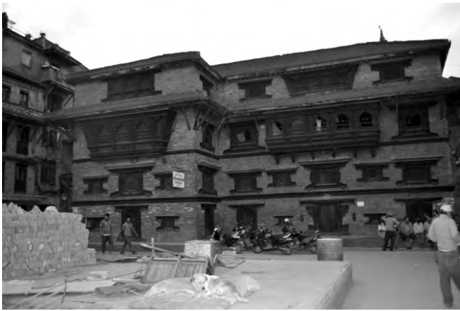
a) Undamaged masonry confined within timber straps, Chamyasingh
