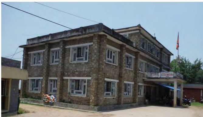
a) A Stone masonry building in cement mortar with RC floor and roof slab
