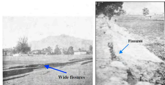
Fig. 12 Liquefaction in Tundhikhel area, Kathmandu by the 1934 earthquake (after Rana, 1935)
