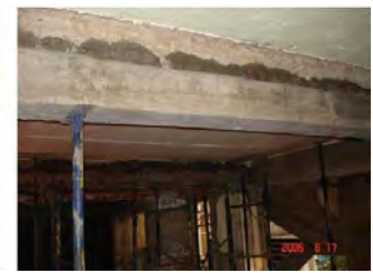
Figure 13. Repair of a beam with micro concrete
