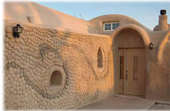
Figure 9: Earthbag house built by Nader Khalili (Turner, I., 2016)
