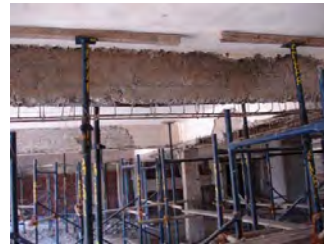
Figure 12. Preparation for micro concrete of a beam
