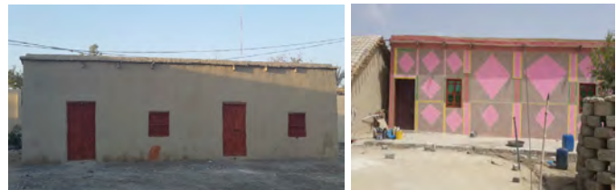
Fig. 5 Views of seismic resistant model houses in Awaran: (a) cob house; (b) CM house
