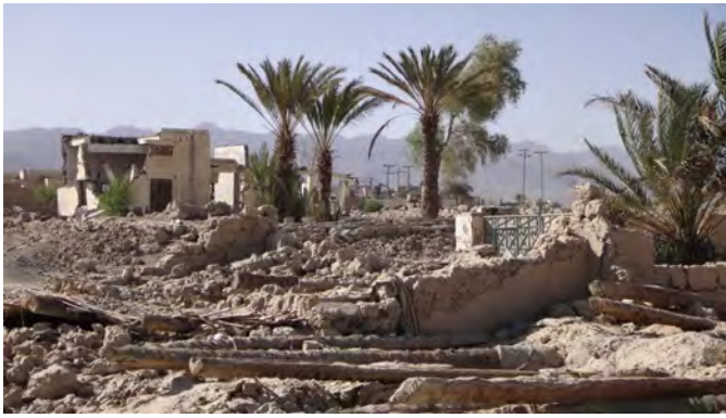
Fig. 3 Damaged buildings in Gajjar
