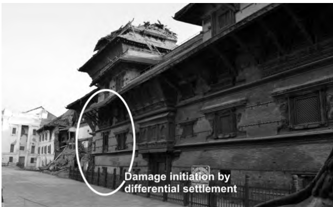
a) Westward view of damaged Basantapur Palace Tower (with Gaddi Baithak partially visible at the left of the photograph), Kathmandu Durbar Square
