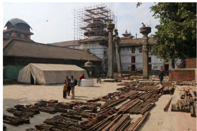
sorting of salvaged wooden elements from Hanuman Dhoka Durbar Square © Kai Weise
