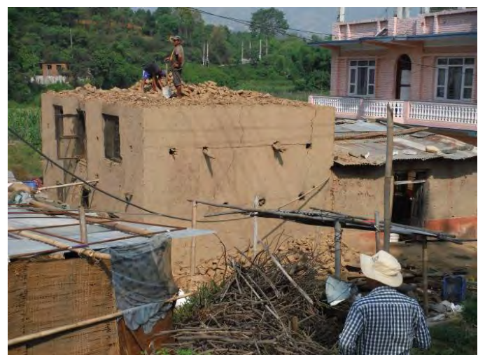
b) An adobe building under partial demolition
