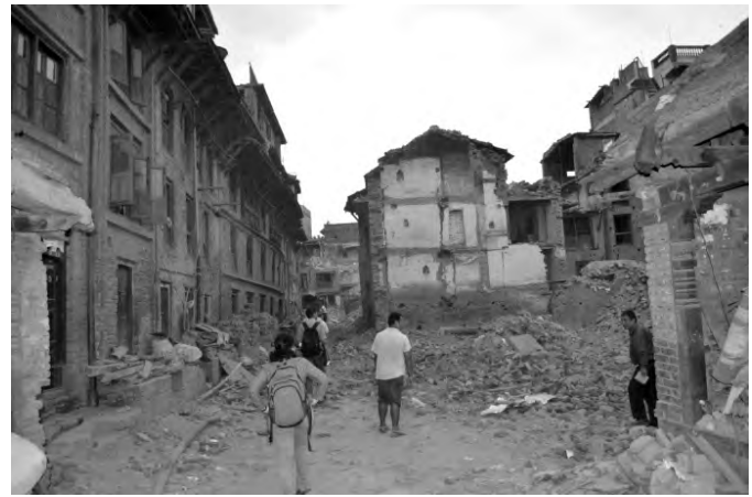
b) Damaged masonry buildings of Chamyasingh
