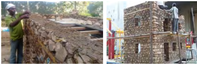
Fig 6 A - 2 1/2 story test model under construction
