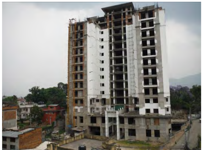
A typical multi-storey RC frame building with masonry infill
