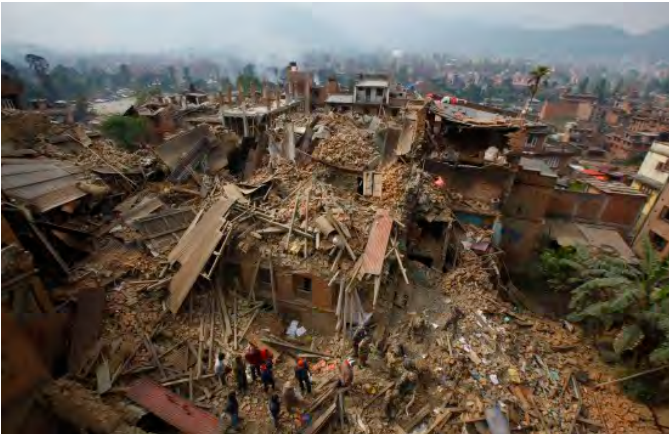
c) Destroyed masonry buildings
