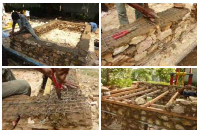
Fig 4 – Construction sequence of 1 1/2 story model
