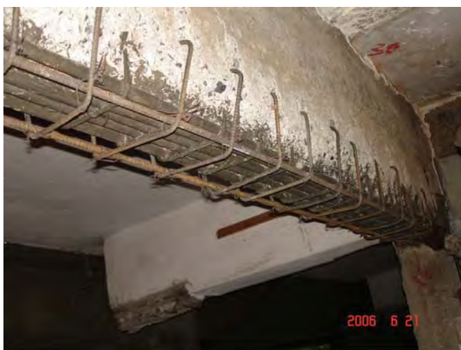
Figure 7. Additional reinforcements and shear connectors provided
