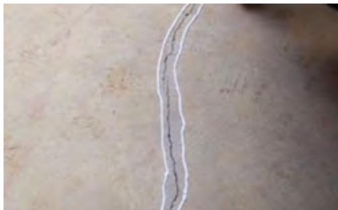
Figure 1. Crack to be filled with ready to use polymeric repair grout
