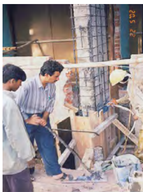
Figure 10. Preparation for micro concrete of a column
