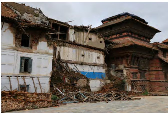
Collapsed structures of the Hanuman Dhoka Palace Museum, Kathmandu © Kai Weise
