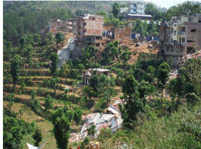
Figure 8: Destruction of buildings on steeply sloping ground.
