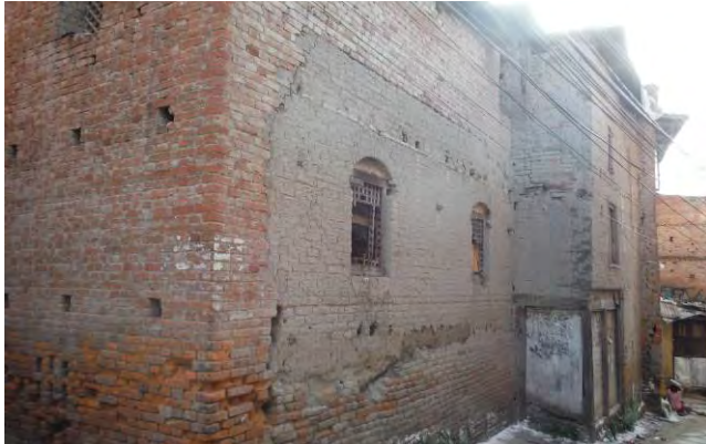
c) Mixed walling materials (adobe and fired brick)
