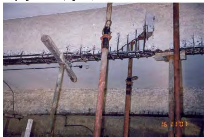
Figure 6. Props for micro concrete
