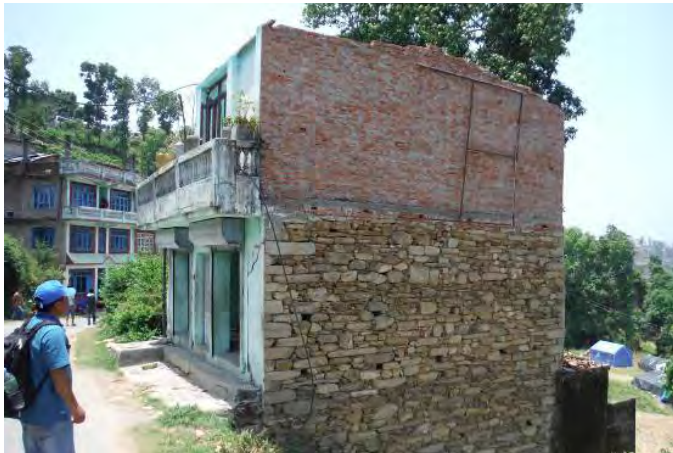
b) Stone and fired brick walls
