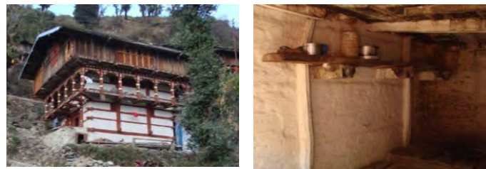
Figure 2 Vertical timber reinforcement in Uttarakhand houses
