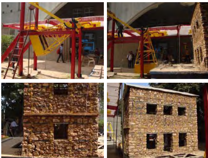
Fig 7 – Impact 14 - Pendulum at 67° inclination; Mortar and stones etc. falling at impact; Diagonal crack at NW base; Stone chips and mud mortar fallen out near S side base
