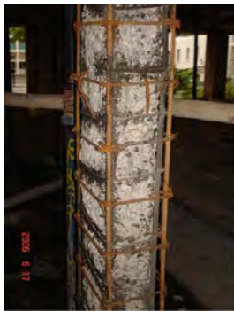
Figure 8. Additional reinforcements provided for jacketing
