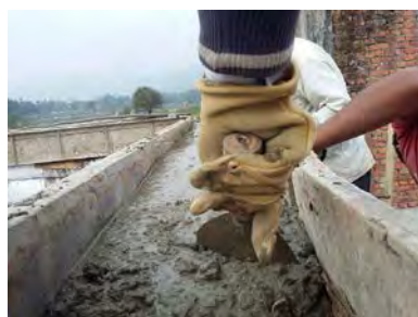
Figure 16: Concrete Bond Beam (Good Earth Nepal, 2015)
