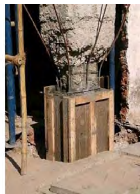
Figure 11. Repair of a column with micro concrete
