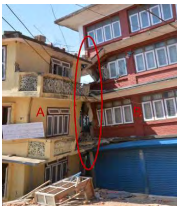
Photo 2: Soft story failure (lost their lower 2 and 4 stories) of buildings in Gongabu
