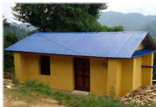
Figure 2: Completed Earthbag House in Gorkha, built by Good Earth Nepal (Good Earth Nepal, 2015).
