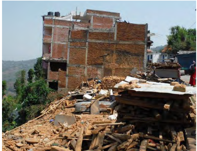
A typical RC frame building on steep terrain
