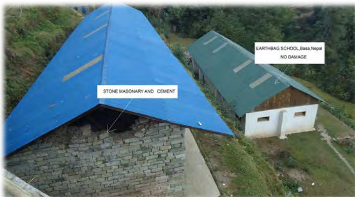
Figure 10: Earthbag School in Basa, Nepal built by Small World next to a damaged stone building (Good Earth Nepal, 2015)
