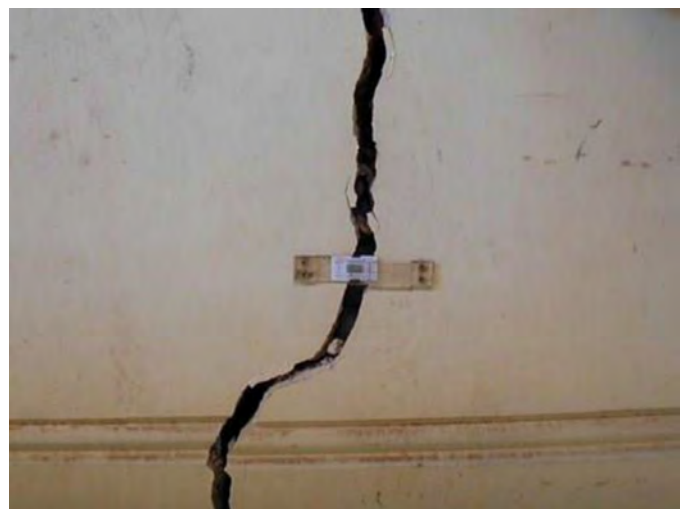
Figure 2. Stitching of cracks in masonry structures
