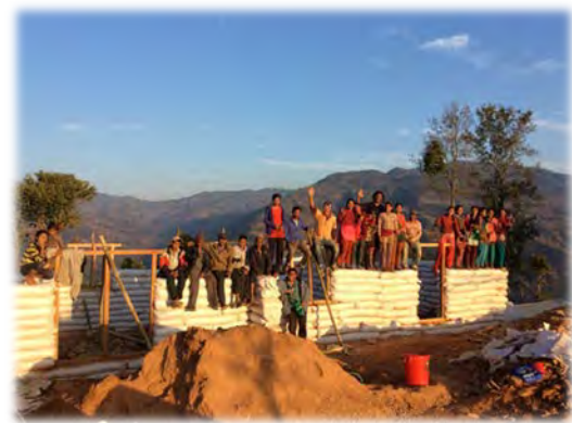
Figure 11: Earthbag School built by First Steps Himalayas survived the earthquake with no damage, Sindhupalchok (Geiger, O., 2013)
