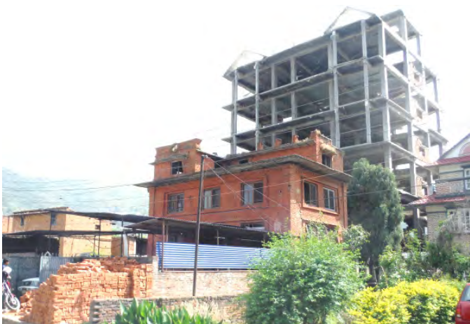
b) A brick in mud mortar with RC slab, Kathmandu valley
